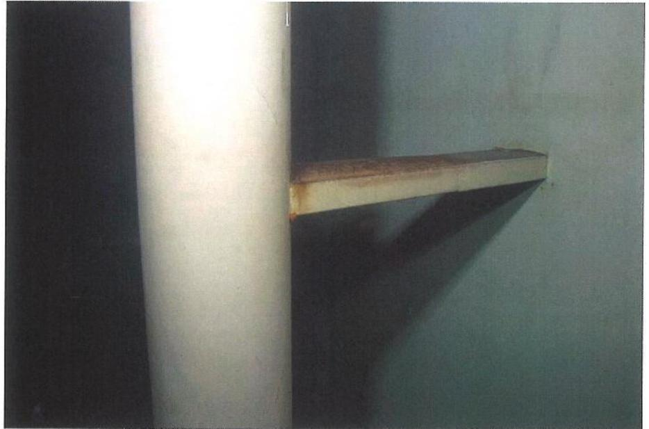
I-28 View of the bottom of the overflow, illustrating generally good condition of the coating system and heavy sediment on the flange and adjacent bottom plates.
