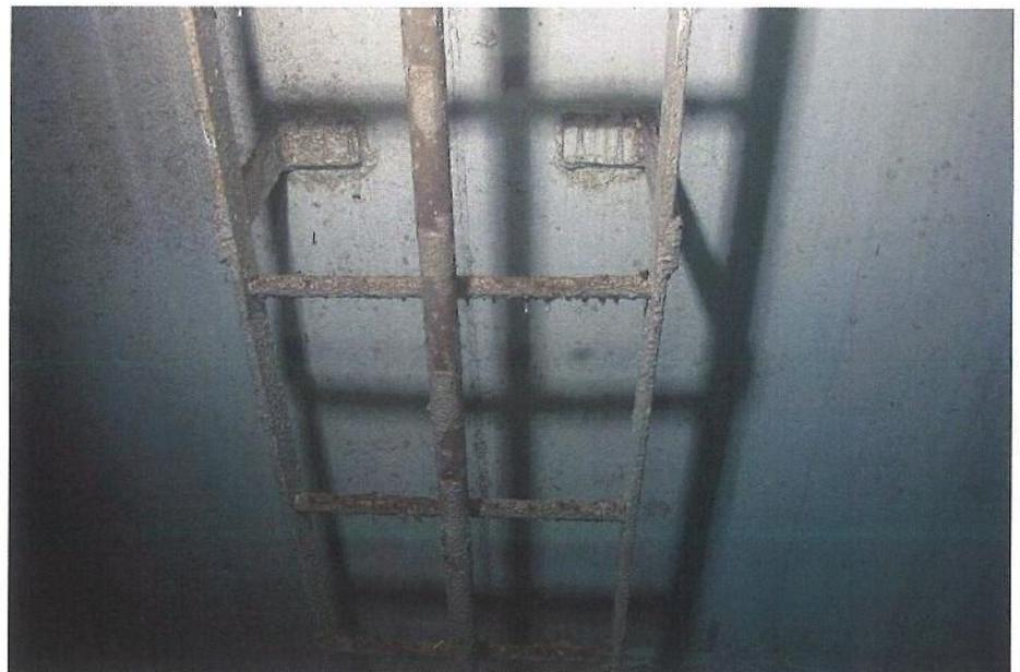
I-20 Same as Photo I-19, except further down the ladder. Note brown sediment on the ladder rungs and adjacent shell and less of the oily substance at this level.
