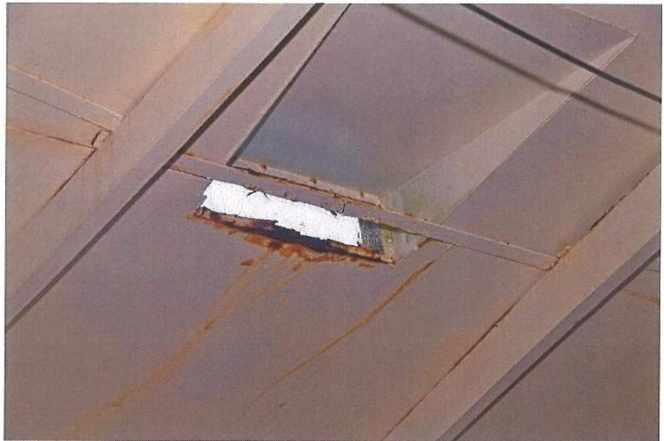
I-13 View of the roof to shell transition, illustrating minor to moderate corrosion along the transition. Note staining running down the shell below the transition.
