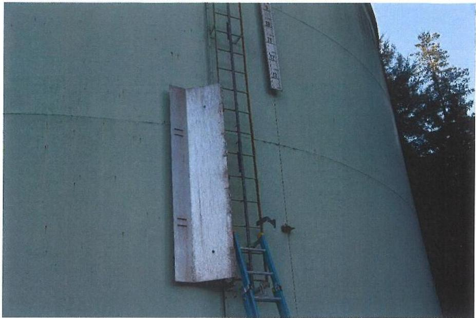
E-18 View of the upper shell courses, illustrating random corrosion along the top angle and spots on the shell.
