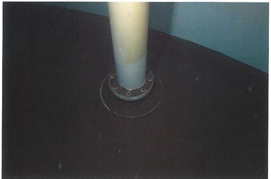
I-29 View of the column, illustrating a spot of corrosion and otherwise generally good condition of the coating system.
