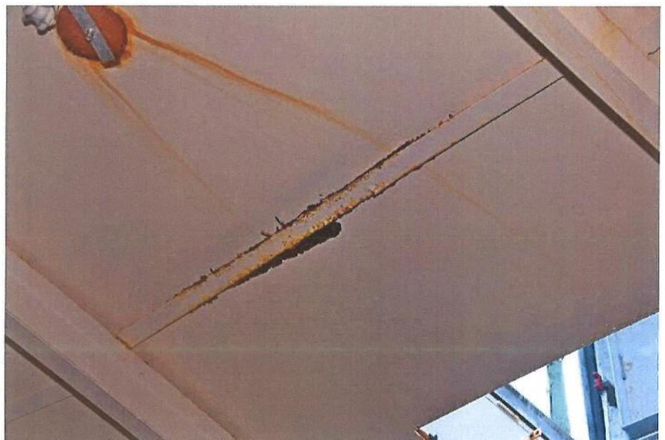
I-8 View of a CP handhole, illustrating cracked and delaminating coating with moderate to severe corrosion around the handhole.
