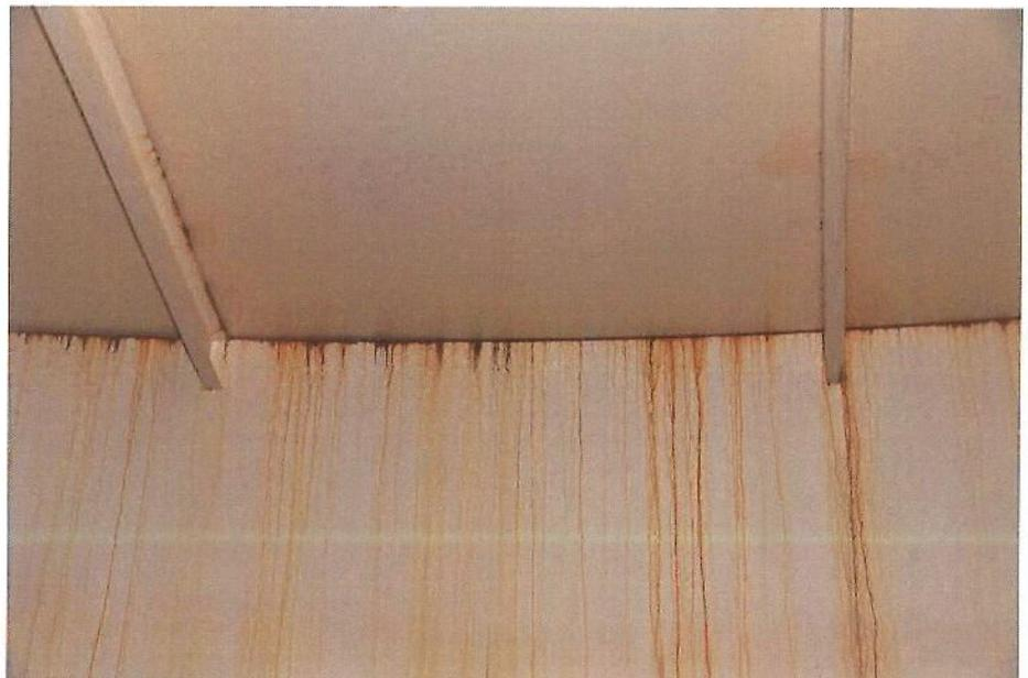
I-14 View of a portion of the shell, illustrating brown staining in the water fluctuation zone and vertical staining below the roof.
