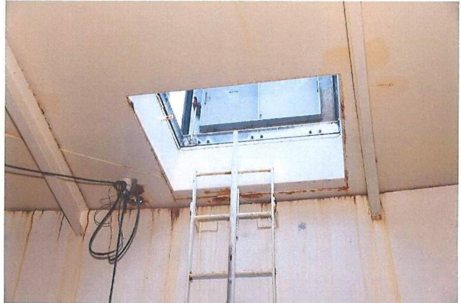
I-19 View of the ladder just below the waterline, illustrating an oily substance on the ladder rungs, side rails, and safety climb rail.
