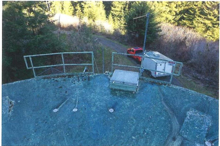
E-13 View of the roof hatch, illustrating generally good condition of the hatch.
