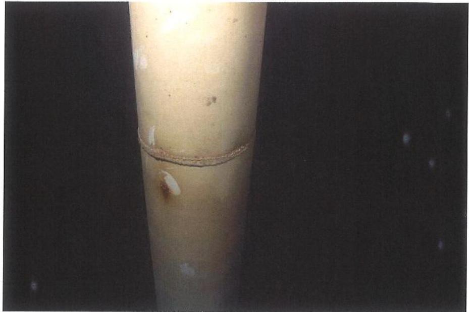
I-30 View of the column base, illustrating dark brown sediment covering all but the edges of the base plate.
