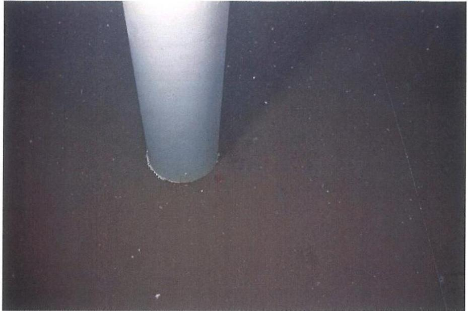
I-33 View of the shell to bottom transition, illustrating good condition of the coating system on the lower shell.
