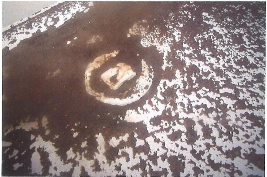
I-37 View of the inlet/outlet pipe and cover, illustrating minor corrosion on the flange below the cover.
