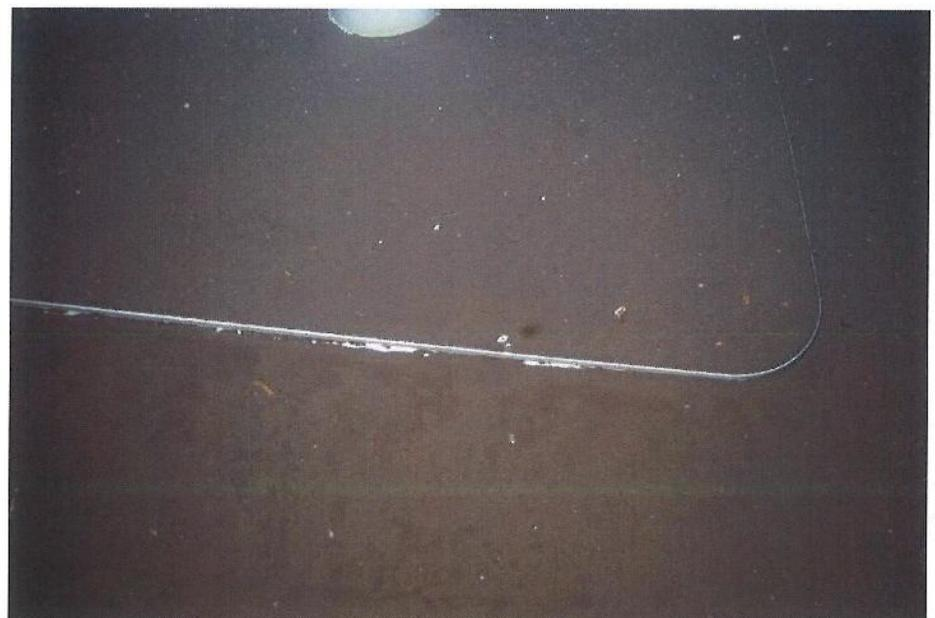
I-32 View of the lower portion of the column, illustrating good condition of the coating system.
