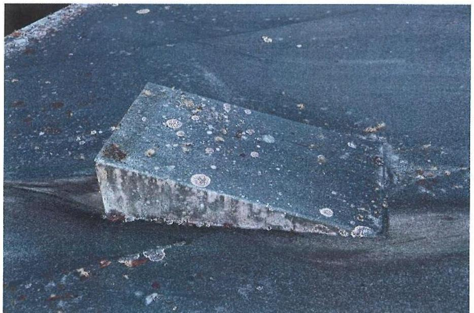
E-8 Same as Photo E-7, except from a different angle. Note moderate to severe corrosion at the perimeter of the vent screen and debris on the roof in front of the vent.
