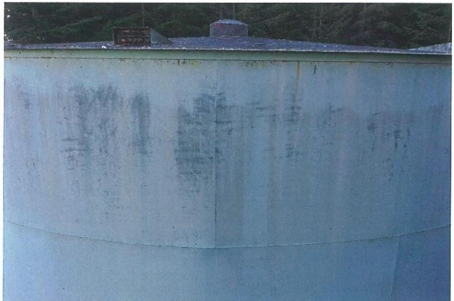
E-19 View of a portion of the shell, illustrating numerous spots of mechanical damage with corrosion.
