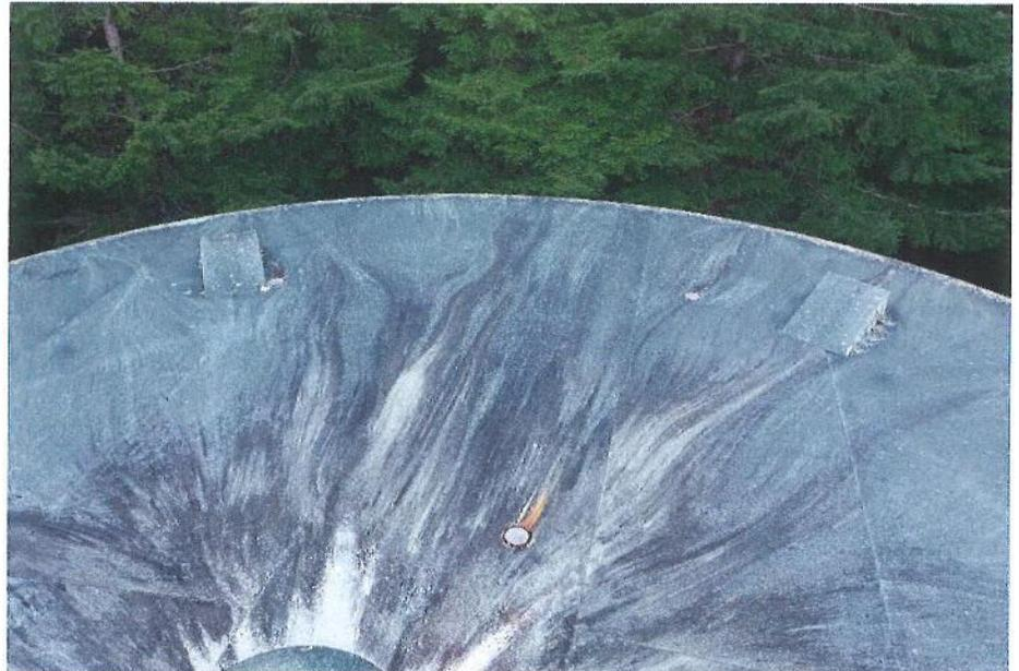
E-7 View of a perimeter vent, illustrating moss covering most surfaces.
