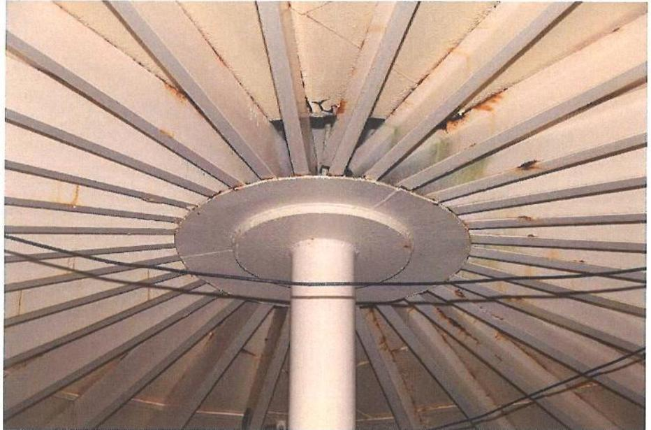
I-4 View of a portion of the roof, illustrating random corrosion and staining at the lateral straps and roof lap joints.
