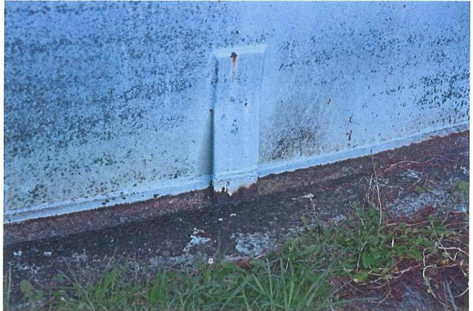
E-25 View of the bottom plate extension (BPE) and two anchor straps, illustrating minor to moderate corrosion along the BPE and bottom of both straps.
