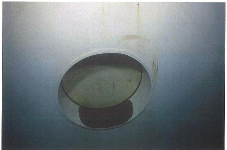
I-26 View of the overflow pipe, illustrating brown staining and an oily substance on the overflow pipe and stand-off bracket.
