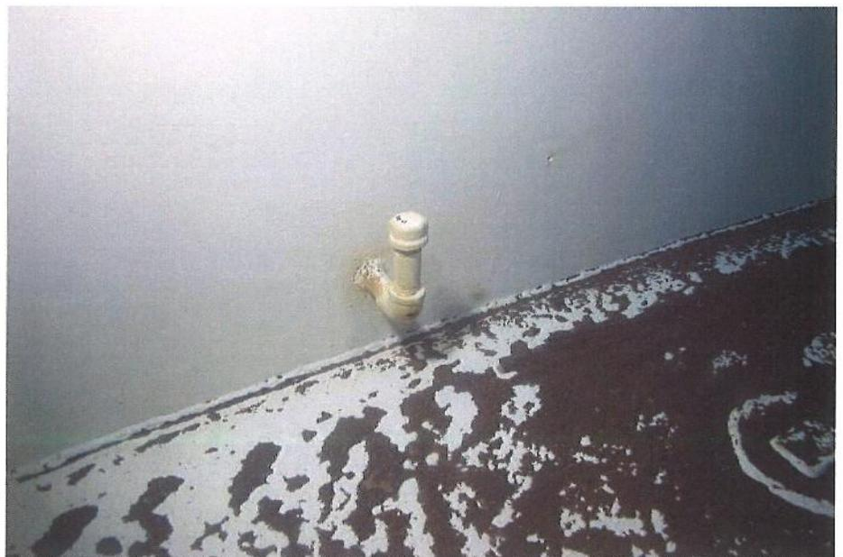
I-35 View of bottom plates, illustrating good condition of the coating system.
