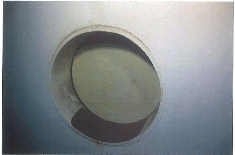
I-25 Same as Photo I-24, except at the other manhole. Note spots of corrosion on the adjacent shell.
