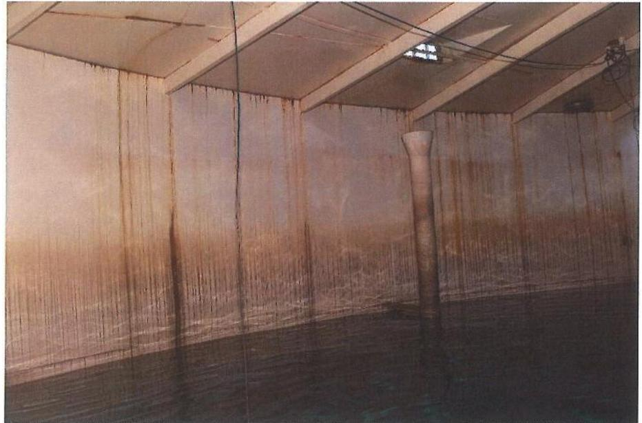
I-16 View of the overflow, illustrating brown staining on the pipe and adjacent shell in the water fluctuation zone.
