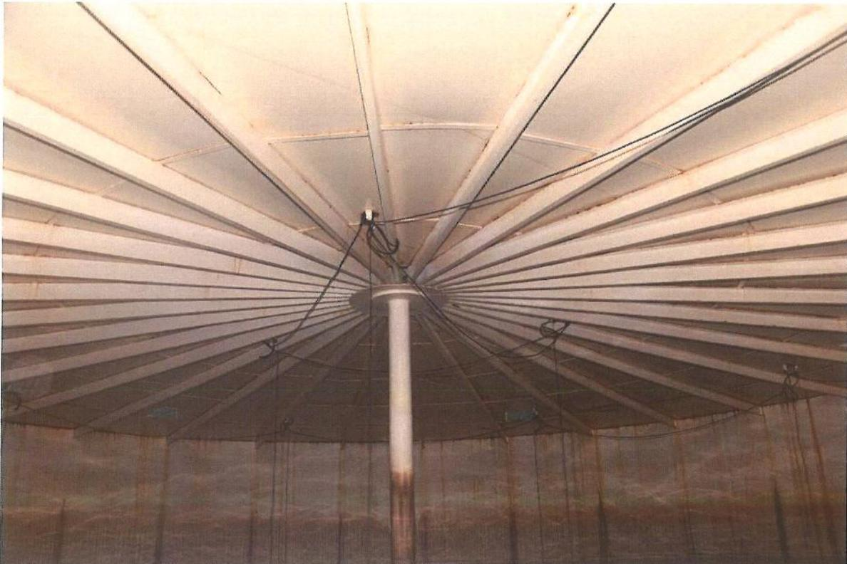
I-2 View of the center support column and rafter ends, illustrating minor corrosion at the edge of the support plate and moderate to severe corrosion along the upper rafter flanges.
