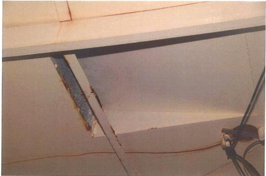
I-12 Same as Photos I-9 through I-11, except at a different vent. Note severe corrosion at the perimeter of this vent.
