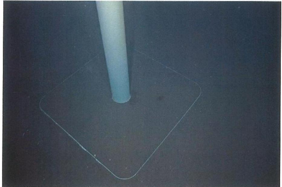
I-31 View of the edge of the base plate, illustrating good condition of the coating system that can be seen.
