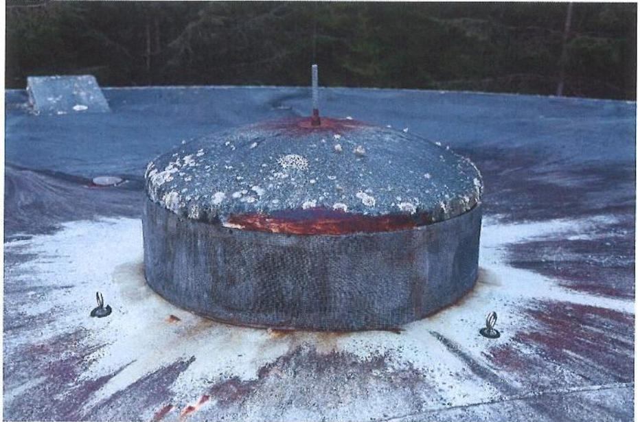
E-4 Same as Photo E-3, except in a different location. Note spot of severe corrosion on the roof.
