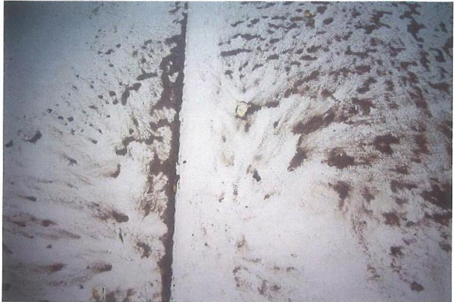
I-36 View of a circular patch plate, illustrating good condition of the coating system that can be seen.
