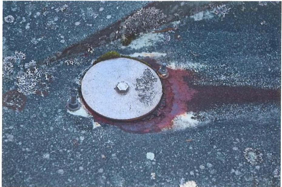
E-12 View of the roof hatch/work area, illustrating moss on all surfaces and otherwise generally fair condition of the paint system.
