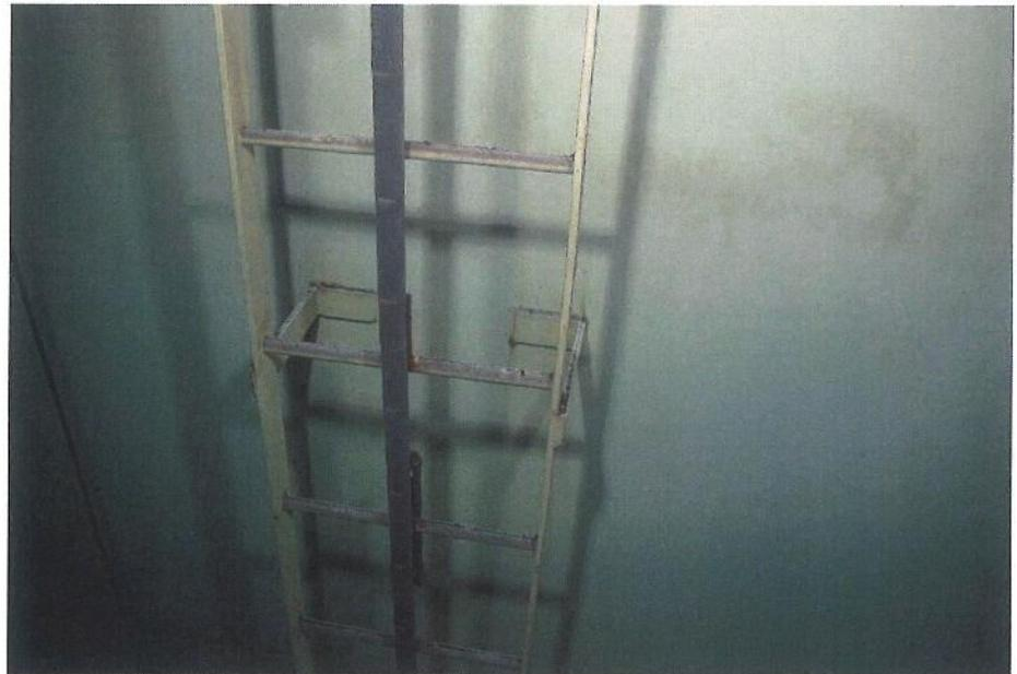
I-22 View of the bottom of the ladder, illustrating minor corrosion at the ends of the rungs and otherwise generally good condition of the coating system.
